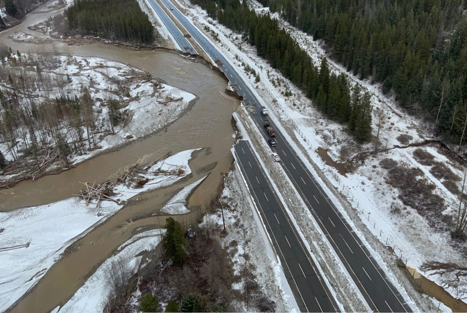
Bank erosion on the Coldwater River, Photo by Carie-Ann Lau
