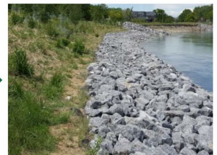
PICTURE 2 Site 4 in 2023, following works.
